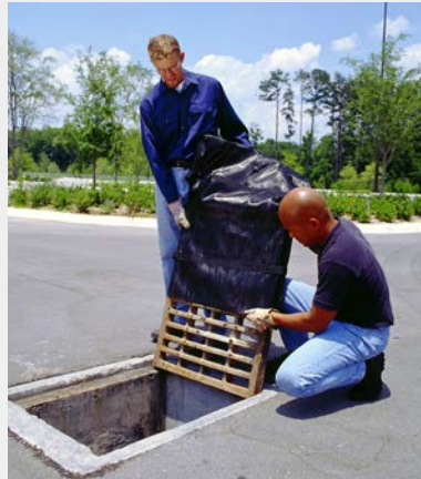
Sampling Port option (Part# 9271) allows use of the Ultra-Universal Sampler (see page 72) to test post-treatment.
